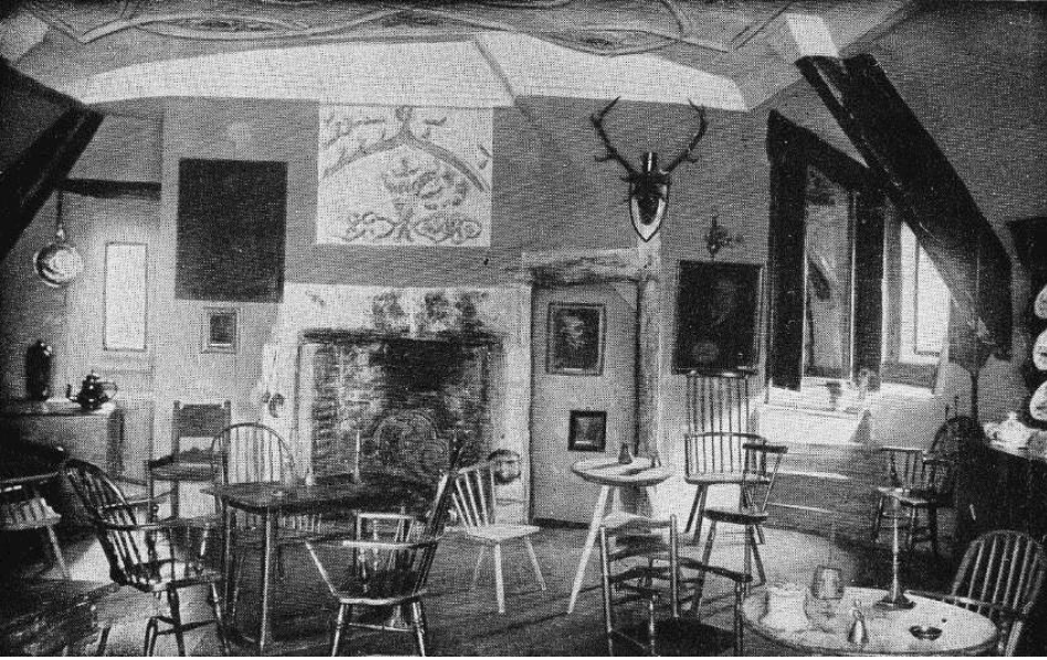
Left: This room is known as the King's Bedchamber, the decorated ceiling can just be seen at the top of this old photo and the decorative plasterwork on the chimney breast. To the right of the fireplace is the entrance door and farther right are stairs leading to the attic. As with the other rooms it has been furnished with antiques and furniture
