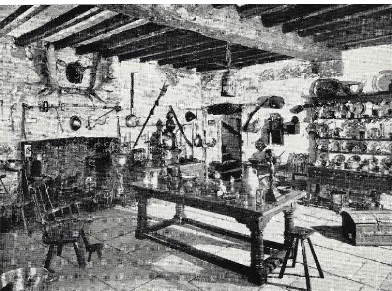
Left: The ground floor showing the original oak beams and stone fireplace with a roasting spit in front. A suit of armour stands to the right of the fireplace. The decorated plasterwork frieze can just be seen below the rafters and above the stone doorway leading to steps to the second floor. This room is filled with a large range of antiques
