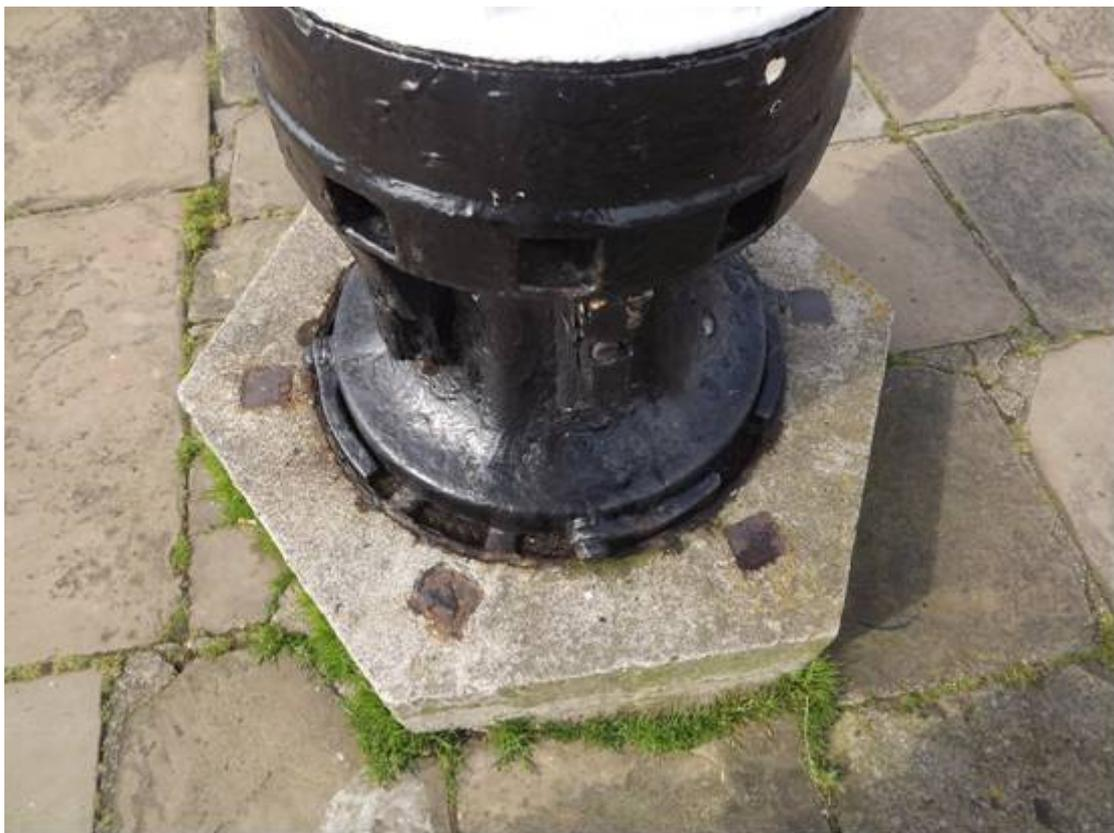
*Plate 71 Vincent's Pier, Lighthouse Pier, detail of base of large capstan, showing pawls and pawl ring forming ratchet mechanism*
