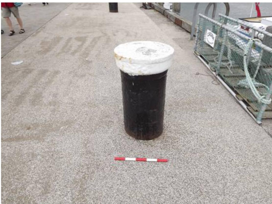
*Plate 44 Vincent's Pier, Type C bollard on 'Old Pier' (1m scale)*
