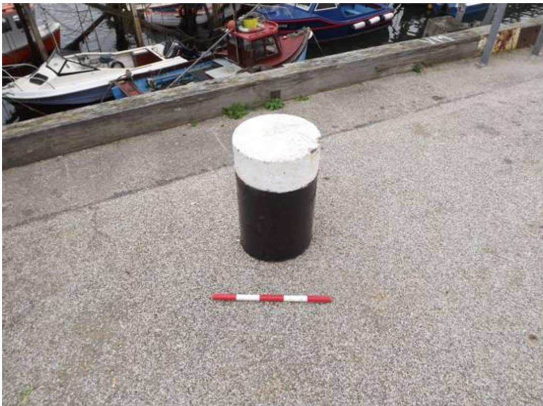
*Plate 45 Vincent's Pier, plain concrete-filled bollard on 'Old Pier' (0.5m scale)*
