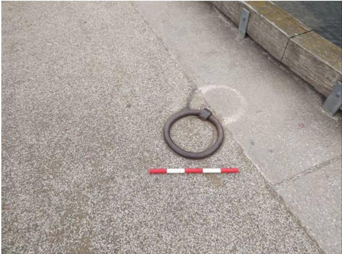
*Plate 47 Vincent's Pier, cast iron mooring ring on 'Old Pier' (0.5m scale)*
