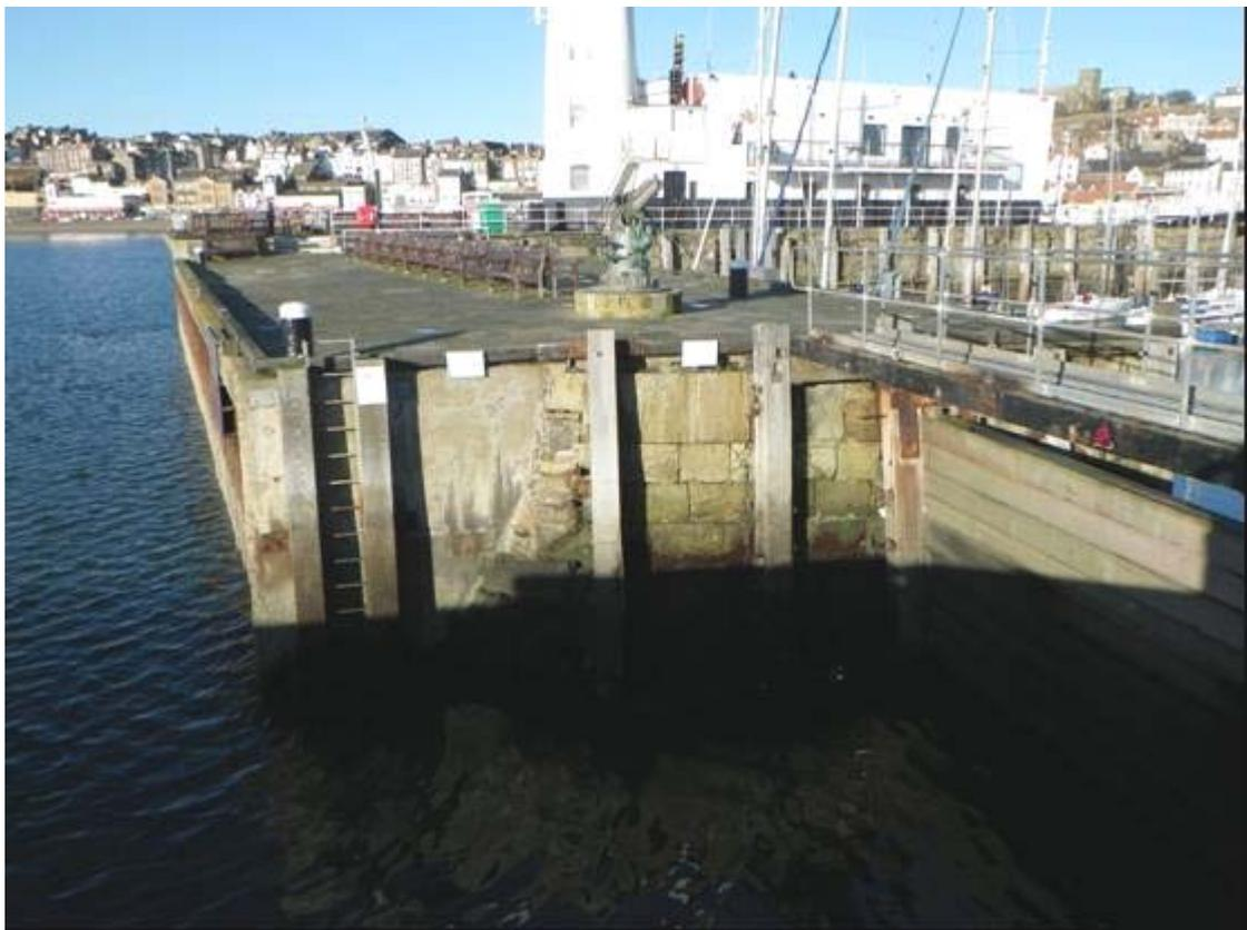
*Plate 52 Vincent's Pier, in January 2013 following construction of temporary footbridge and insertion of timber stop planks across inner harbour entrance*
