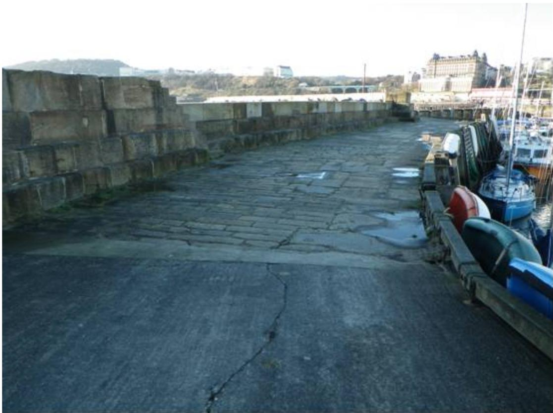
*Plate 18 East Pier, southern section, detail of junction of concrete and stone surfacing, looking south-west*
