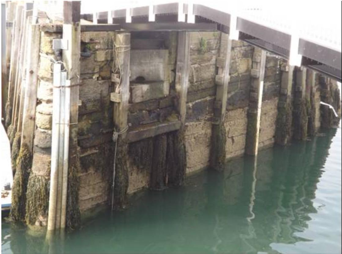
*Plate 39 Vincent's Pier, position of south end of earlier drawbridge visible on island pier below present bridge, looking south-west*
