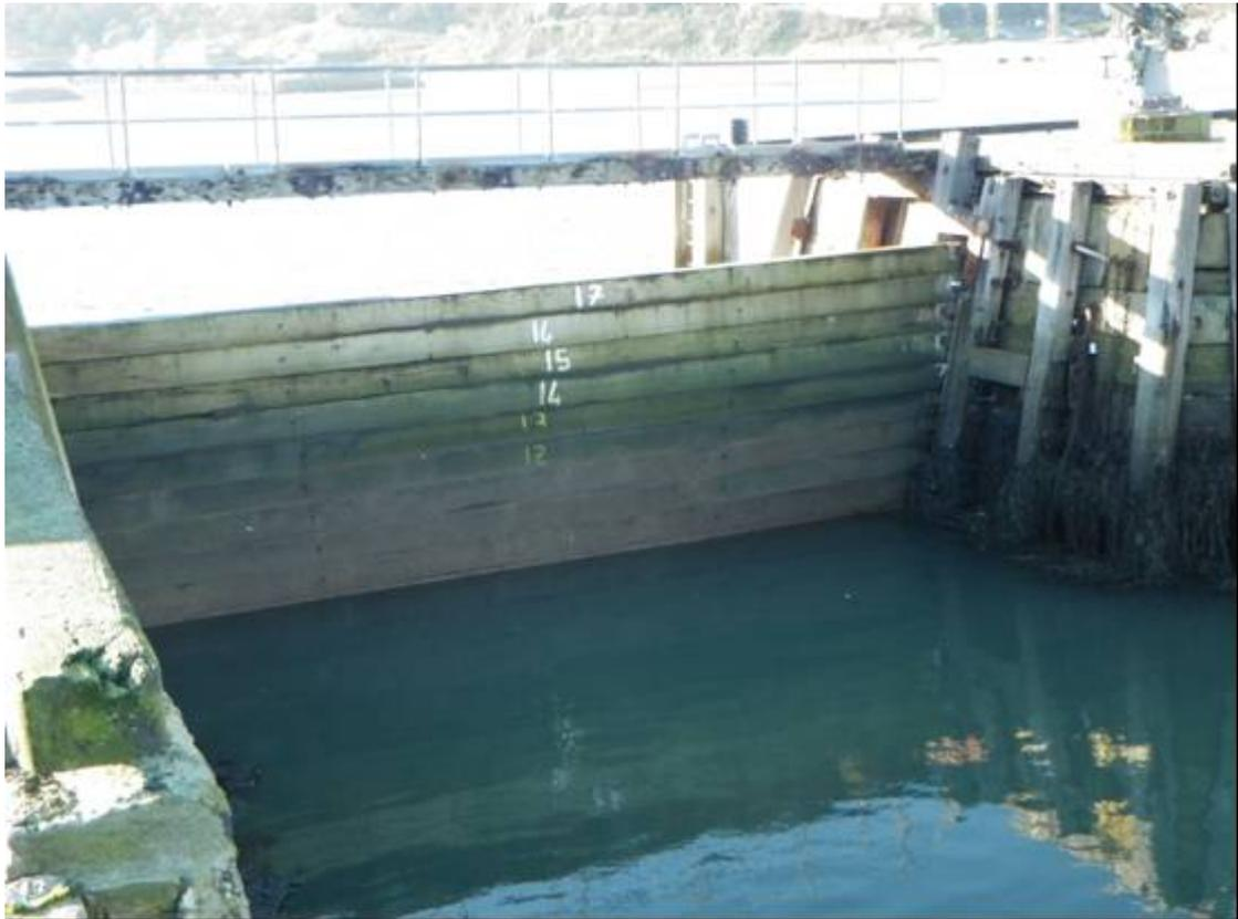
*Plate 53 Vincent's Pier, detail of outer harbour entrance with stop planks and temporary footbridge*
