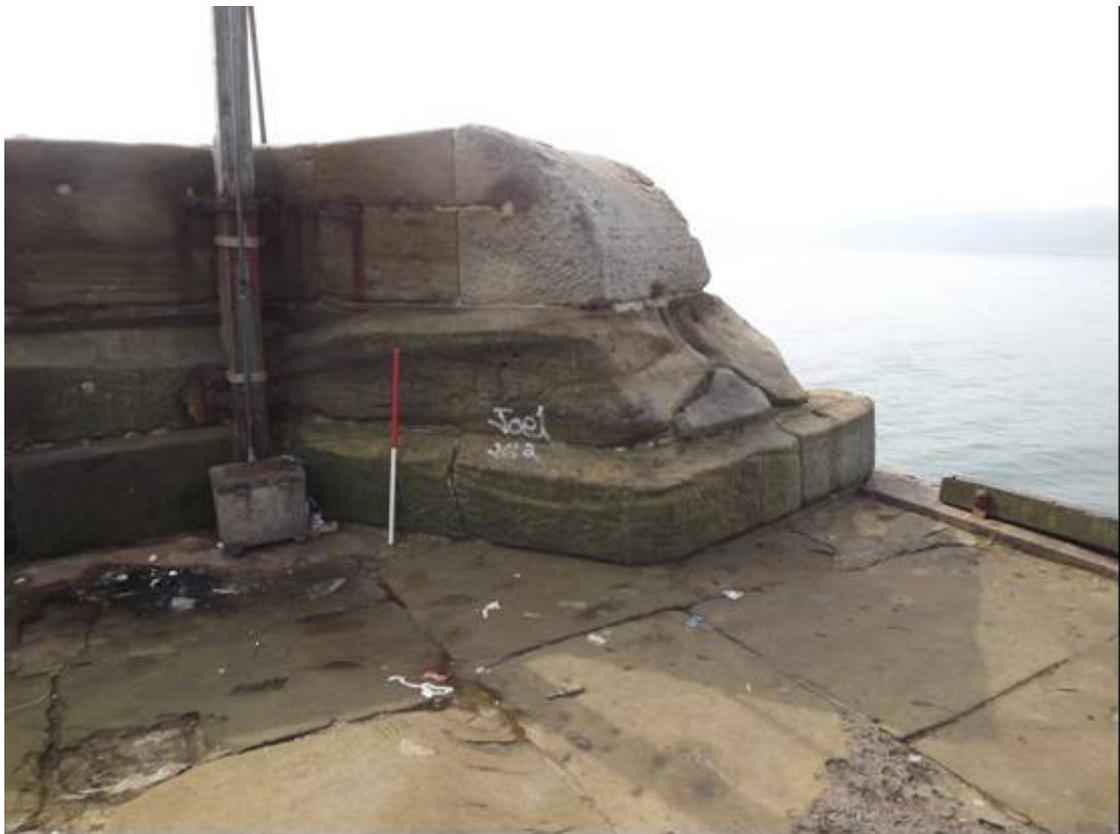
*Plate 24 East Pier, detail of shaped end of original parapet (1m scale)*
