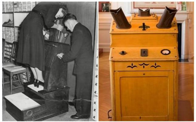
The X-Ray machine known as a fluoroscope used to measure shoe sizes. Courtesy of ORAU
