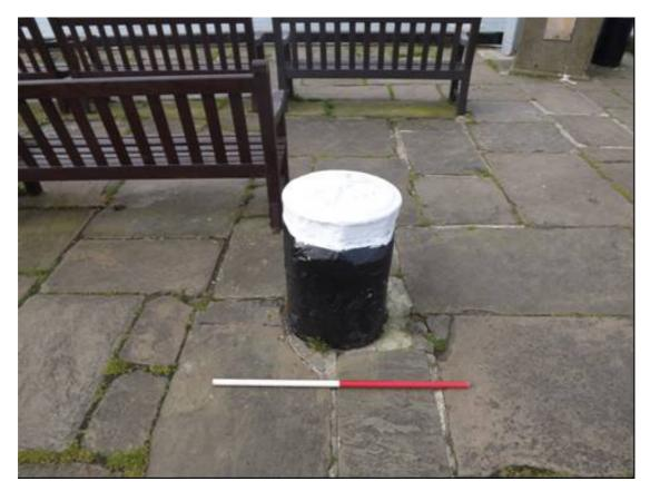
Plate 66 Vincent's Pier, Lighthouse Pier, modified wooden bollard with decorative iron cap (1m scale)
