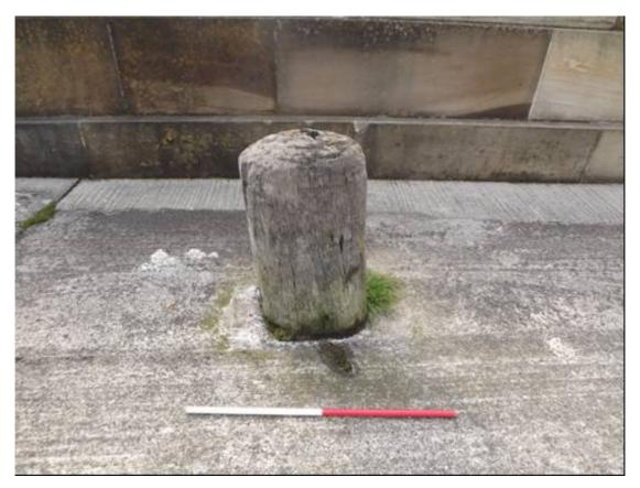
Plate 28 East Pier, Type F wooden bollard (1m scale)
