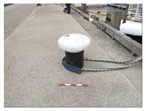
Plate 43 Vincent's Pier, Type B bollard on 'Old Pier' (0.5m scale)
