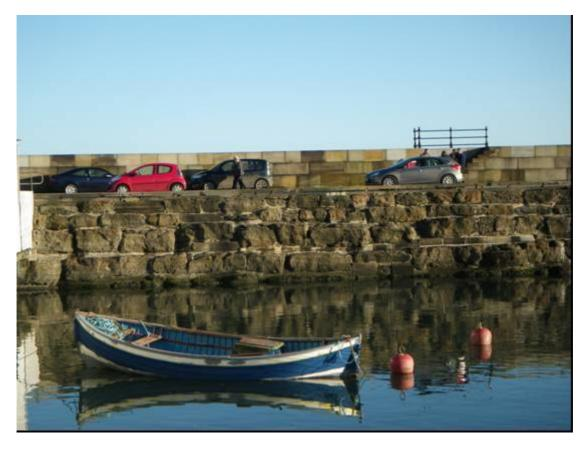
Plate 3 East Pier, inner face of northern section next to Luna Park, showing stone blocks decreasing in size towards top, and northern part of new parapet, looking east
