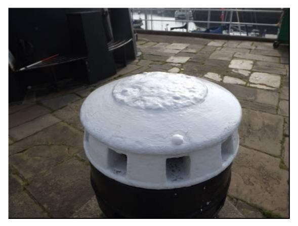
Plate 72 Vincent's Pier, Lighthouse Pier, detail of large capstan head, showing upper row of sockets for capstan bars and corrosion on cap
