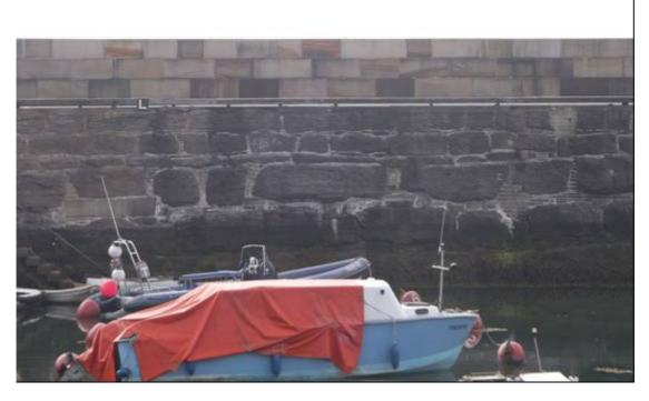
Plate 7 East Pier, detail of inner face, showing extensive patching between original blocks and new parapet, looking south-east
