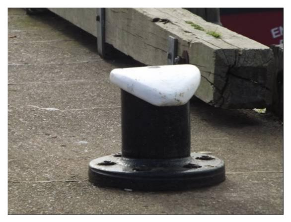
Plate 90 North Wharf, smaller modern bollard with circular baseplate
