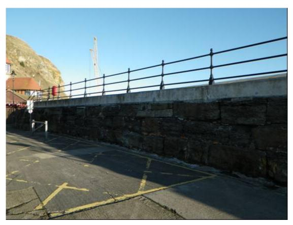
Plate 12 East Pier, original parapet at north end of pier with later cast iron railings, looking north-east
