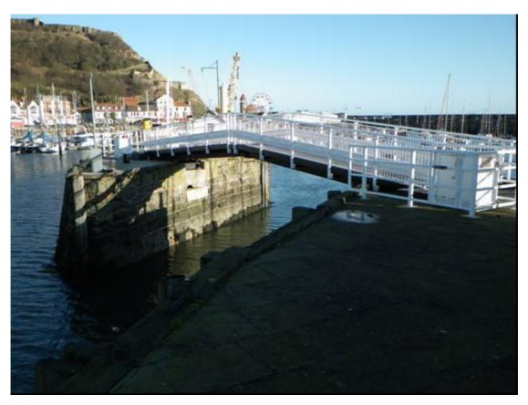
Plate 38 Vincent's Pier, 'Captain Sydney Smith Bridge', looking north-east towards 'Old Pier', position of north end of earlier drawbridge visible directly beneath
