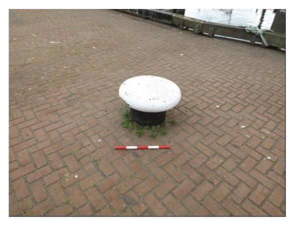
Plate 83 North Wharf, detail of Type B bollard, partly sunk in modern setts (0.5m scale)
