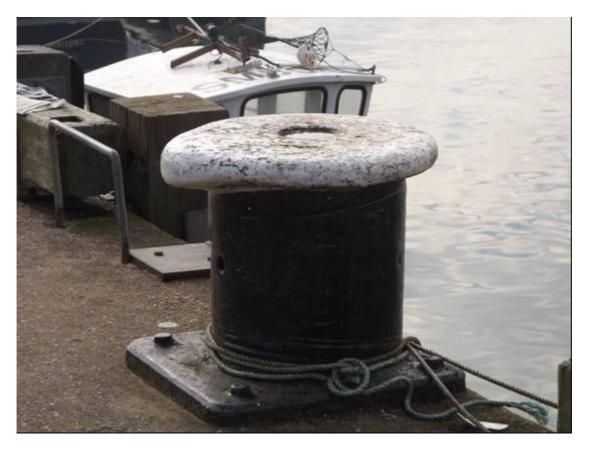
Plate 89 North Wharf, large modern bollard with square baseplate
