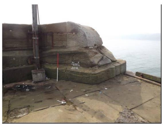
Plate 24 East Pier, detail of shaped end of original parapet (1m scale)
