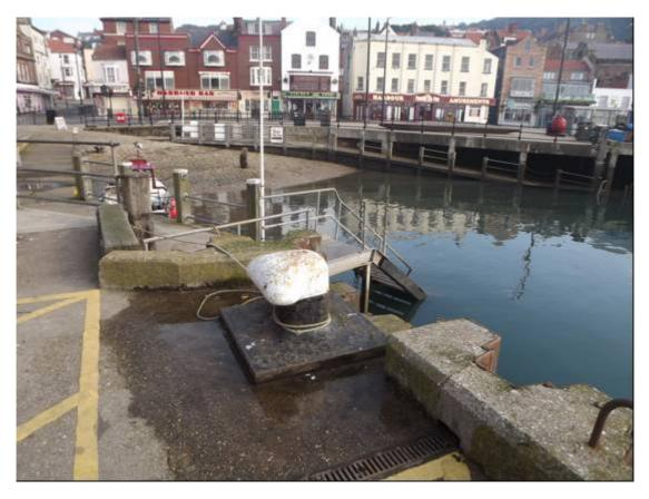
Plate 116 West Pier, modern hammerhead bollard on east side of pier (1m scale), looking north across western slipway to North Wharf
