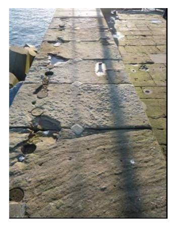
Plate 17 East Pier, southern section, detail of top of original parapet, showing blocked circular sockets for removed cast iron railings
