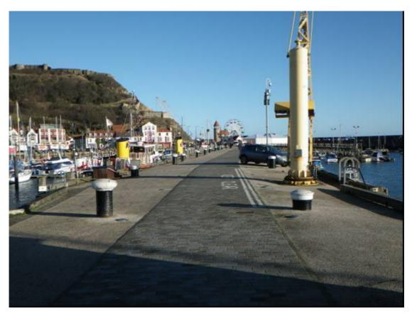
Plate 42 Vincent's Pier, general view along 'Old Pier', with Type B bollard (left) and Type C (right) in front of modern crane, looking north-east
