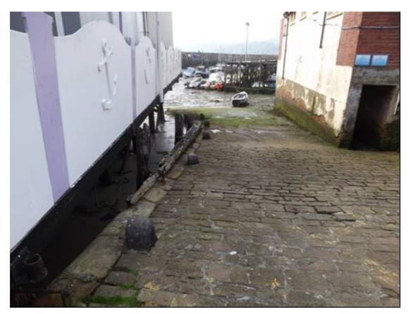
Plate 32 Sandside, slipway east of Vincent's Pier, showing stone posts marking edge, looking south
