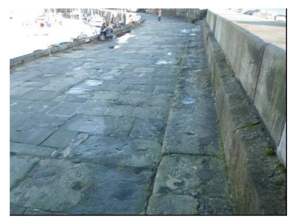
Plate 21 East Pier, showing stone block surface and new section of parapet at south end raised to accommodate rock armour
