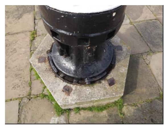
Plate 71 Vincent's Pier, Lighthouse Pier, detail of base of large capstan, showing pawls and pawl ring forming ratchet mechanism
