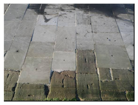
Plate 20 East Pier, repairs to stone surface, showing use of three-legged (rectangular) and split-pin (circular) forms of lewis on old and new sections
