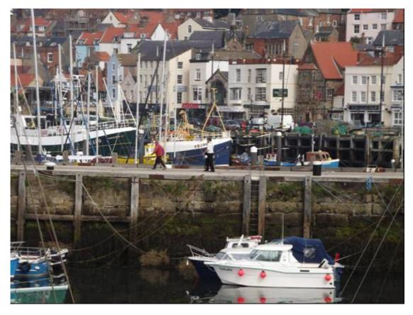
Plate 35 Vincent's Pier, detail of east side of 'Old Pier' showing change in construction between Vincent's work (left) and an existing section, looking north-west
