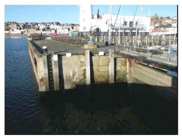
*Plate 52 Vincent's Pier, in January 2013 following construction of temporary footbridge and insertion of timber stop planks across inner harbour entrance*
