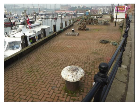
Plate 82 North Wharf, section of rebuilt wharf east of central slipway with Type B bollard and modern setts
