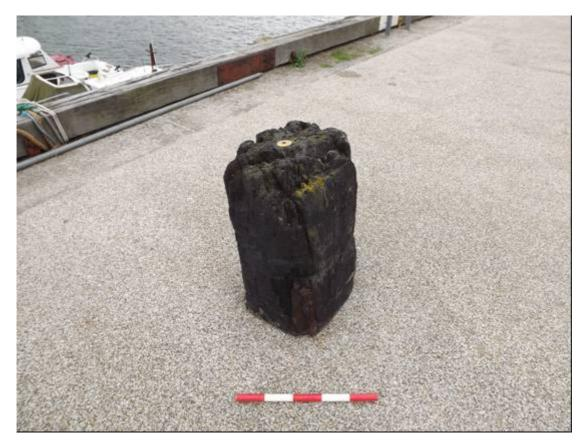
Plate 46 Vincent's Pier, wooden Type D bollard on 'Old Pier' (0.5m scale)
