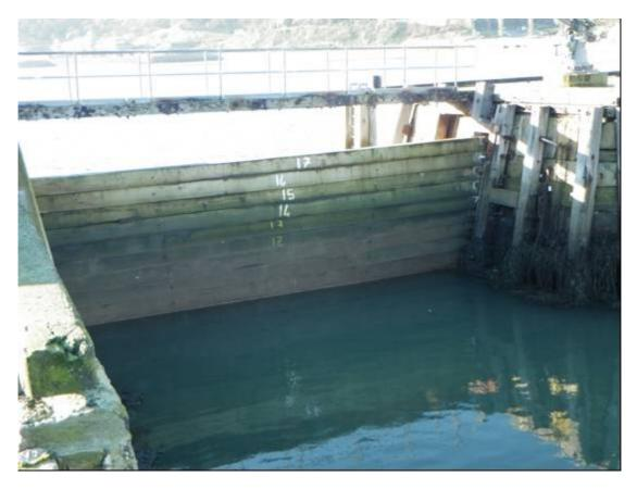
Plate 53 Vincent's Pier, detail of outer harbour entrance with stop planks and temporary footbridge
