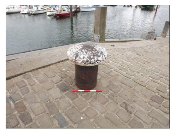
Plate 85 North Wharf, Type B bollard at top of central slipway (0.5m scale)
