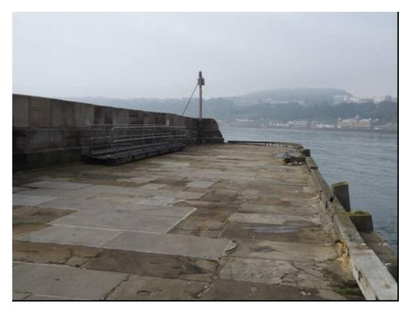
Plate 23 East Pier, original surface and parapet at south end, with temporary bridge stored ready for use, looking south-west
