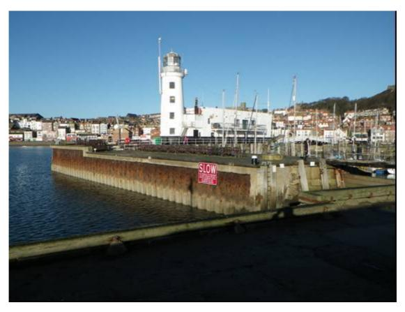
Plate 50 Vincent's Pier, south face of Lighthouse Pier, showing modern steel sheet and concrete refacing, looking north-west
