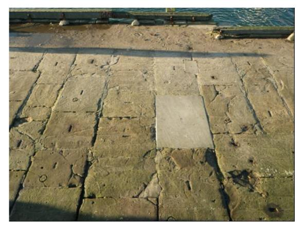
Plate 19 East Pier, stone blocks forming surface of southern section, showing lewis holes, with modern replacement
