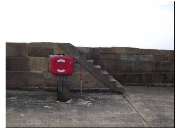
Plate 26 East Pier, Type E wooden bollard next to rebuilt steps to original parapet (1m scale)
