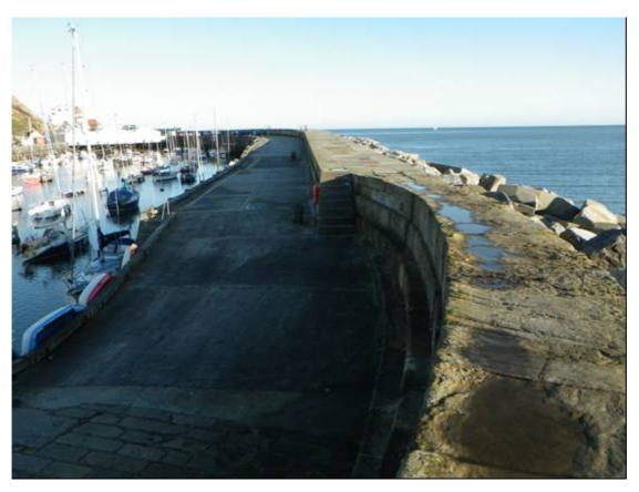
Plate 14 East Pier, junction of original southern section of parapet (foreground) with new central section beyond steps, looking north-east
