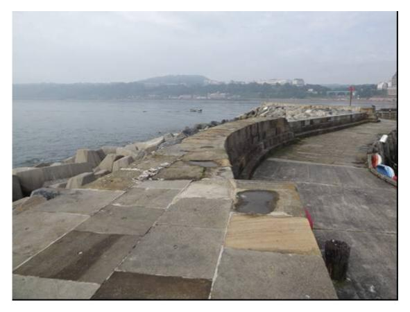
Plate 15 East Pier, southern section, junction of new and old parapets, with rock armour against east face
